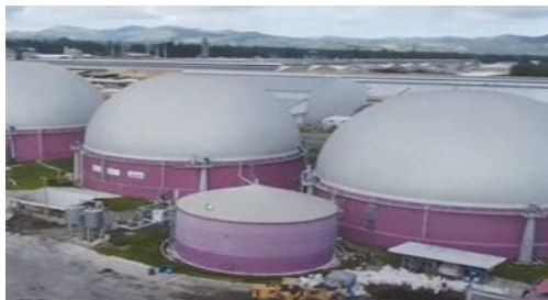
Biogas Power Generation, ITOCHU Corporation, Philippines
