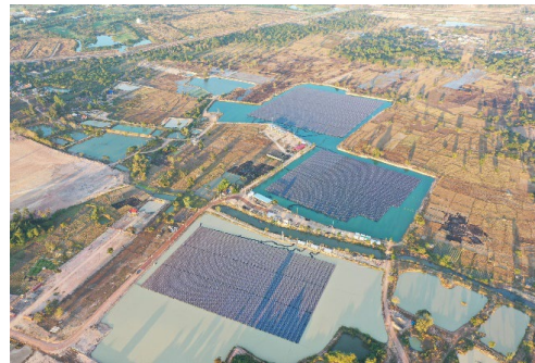
Floating Solar PV, TSB Co., Ltd., Thailand
